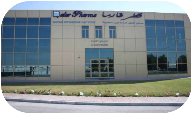
Qatar Pharma Medical Ware house
