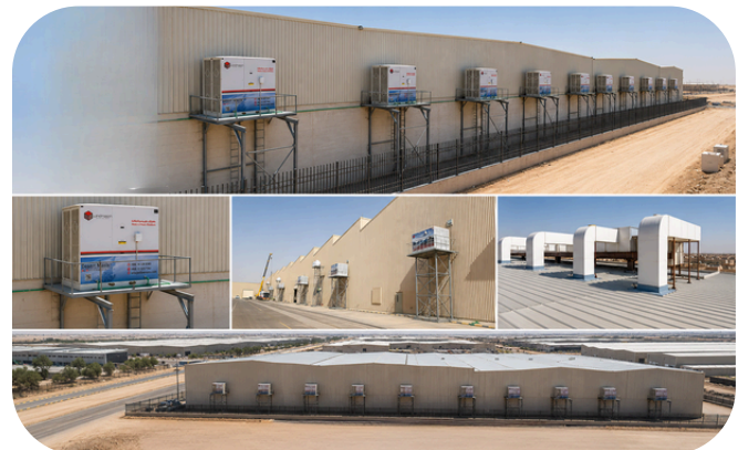
Project: Saudi Railway Workshop in Riyadh مشروع قطار الرياض
