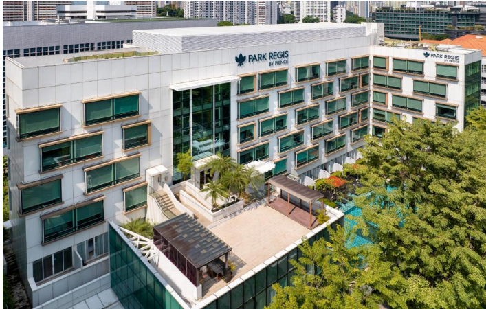
Project: Park Regis Eco Edge AI Deployment for Energy Saving.
