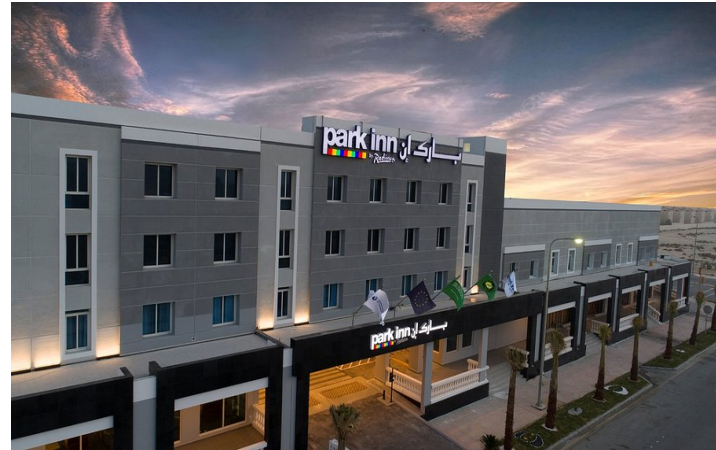
Project: Park Inn by Radisson Eco Edge AI Deployment for Energy Saving.
